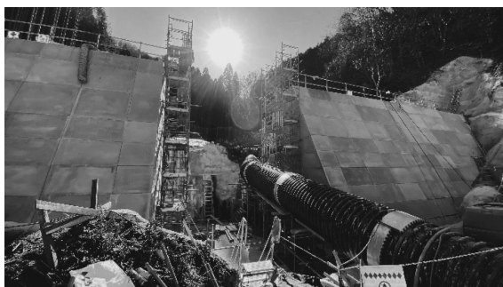
Fig. 2 A check dam constructed after the 2019 Heavy Rainfall Disaster
